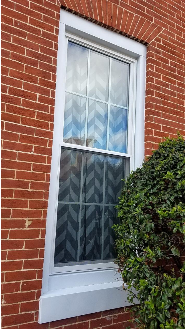
Image 8: 105 Warren Avenue – Detail, newly installed vinyl window, April 2, 2021
